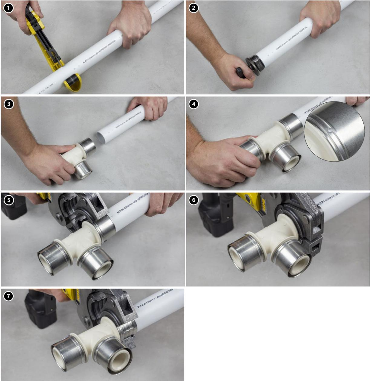
1. Using a pipe cutter for PERTAL pipes or a pipe roller cutter, cut the pipe perpendicularly to its axis at the required length.
