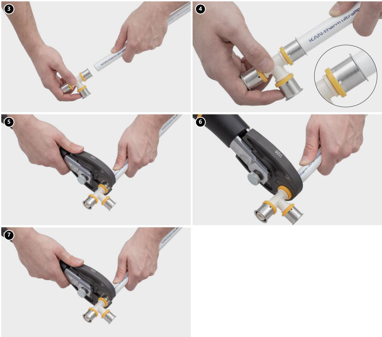
3. Slide the pipe into the fitting until it stops – axis mount of the pipe on the stub of the fitting is required. Check the depth of the fit – the edge of the pipe must be visible in inspection holes.
