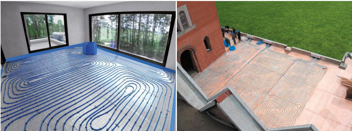
Wet laid floor heating/cooling – pipes embedded in a cast screed
