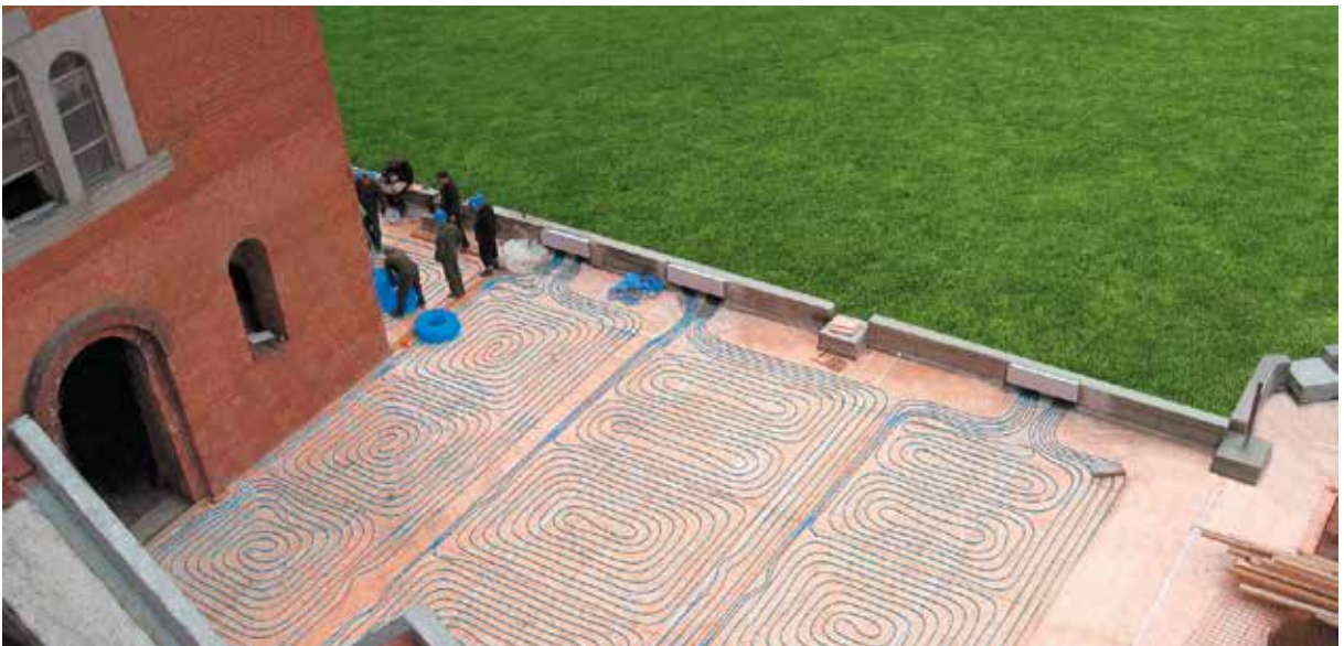
Fig. 5. Heating installation of outdoor patio employing KAN-therm system bluePERT pipes.
