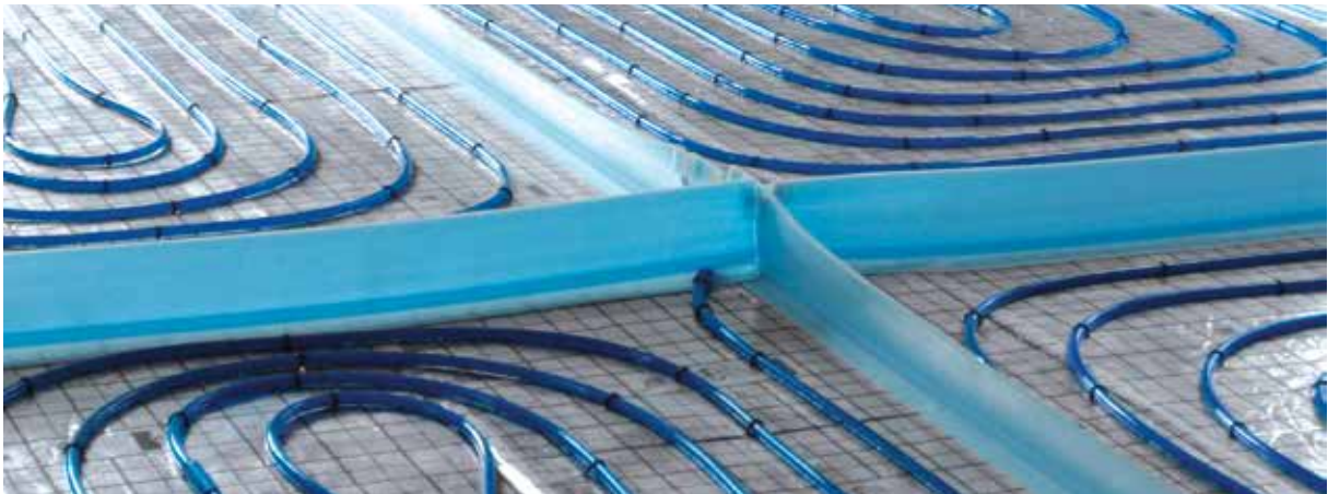
Fig. 14. Distribution of heating fields with dilatation gaps
