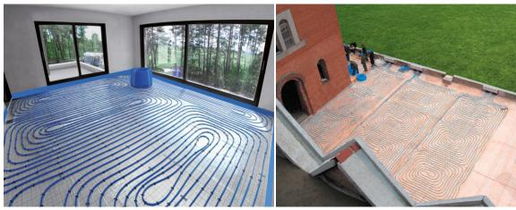
Wet laid floor heating/cooling - pipes embedded in a cast screed
