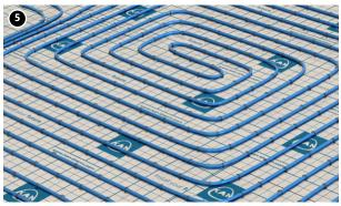
5. Perform a pressure test of arranged coils leakage in accordance with the rules applicable for the surface heating (see section Acceptance forms). After the test, leave the pipes under pressure (min 3 bars).
